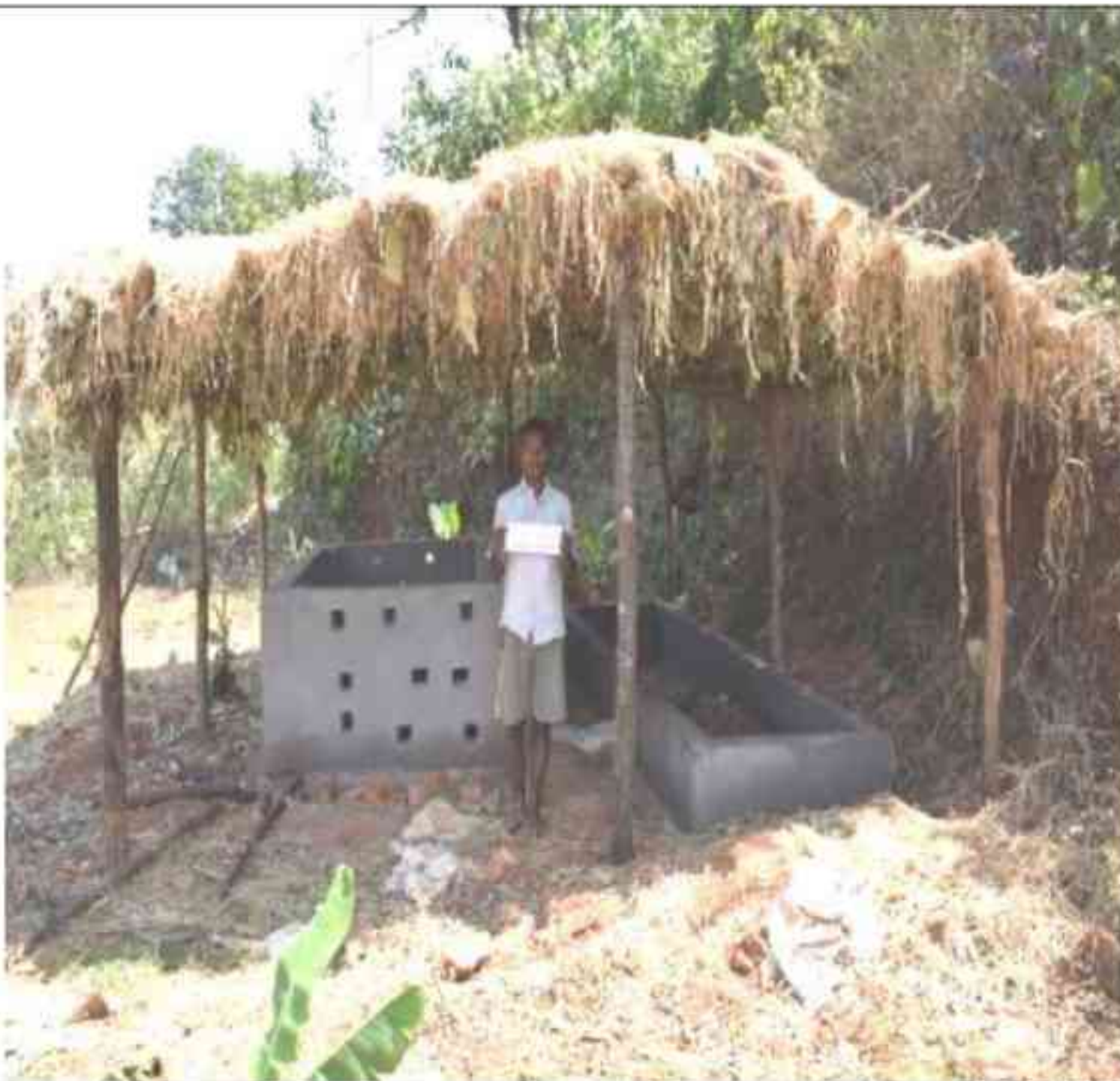
Construction of NADEP and vermin-compost pit
