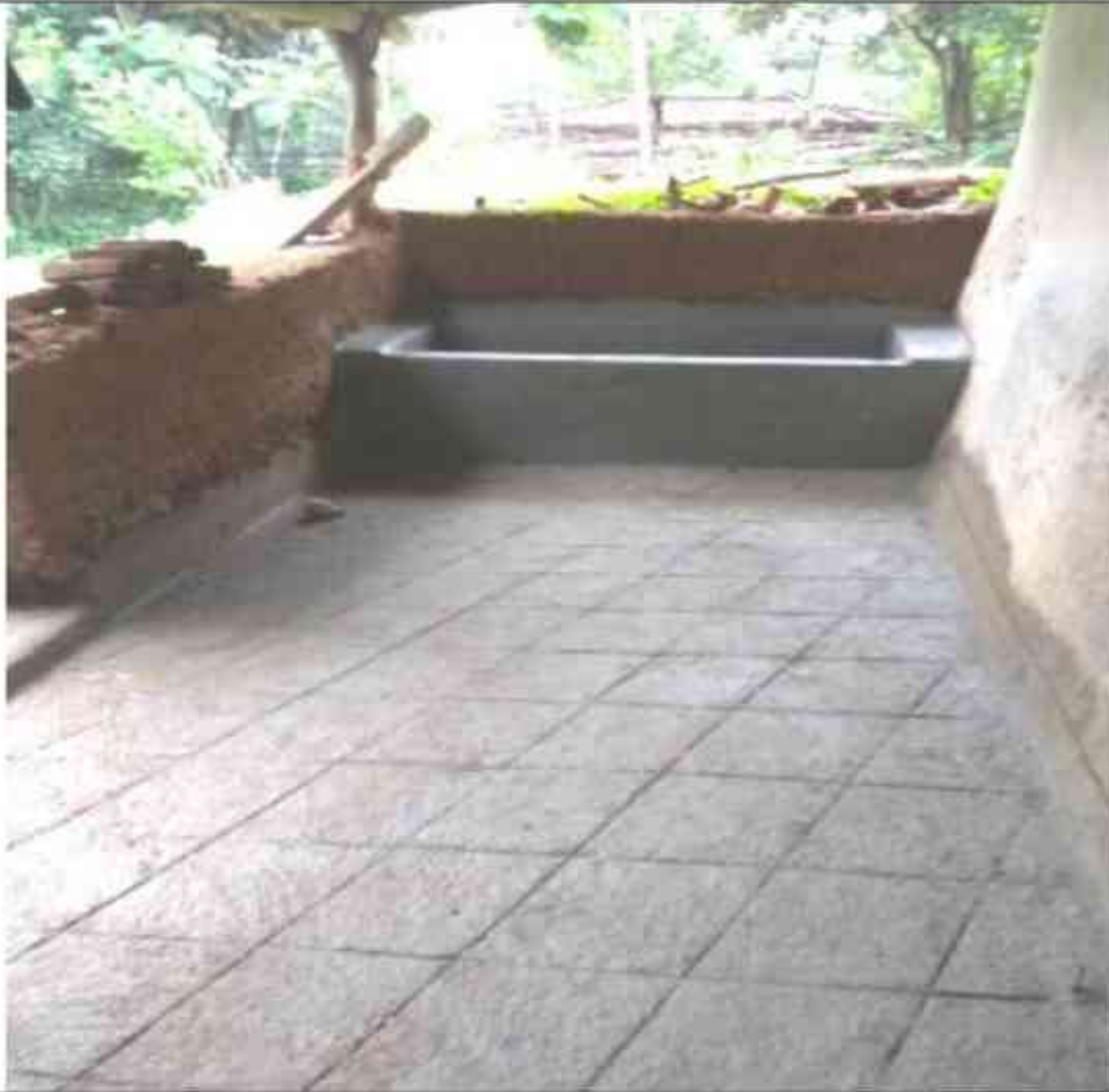
Construction of cow shade floor
